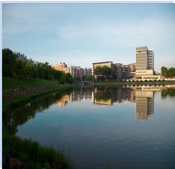
Alexandra Health Cluster- Water from the adjacent Yishun pond is used to irrigate the gardens.
